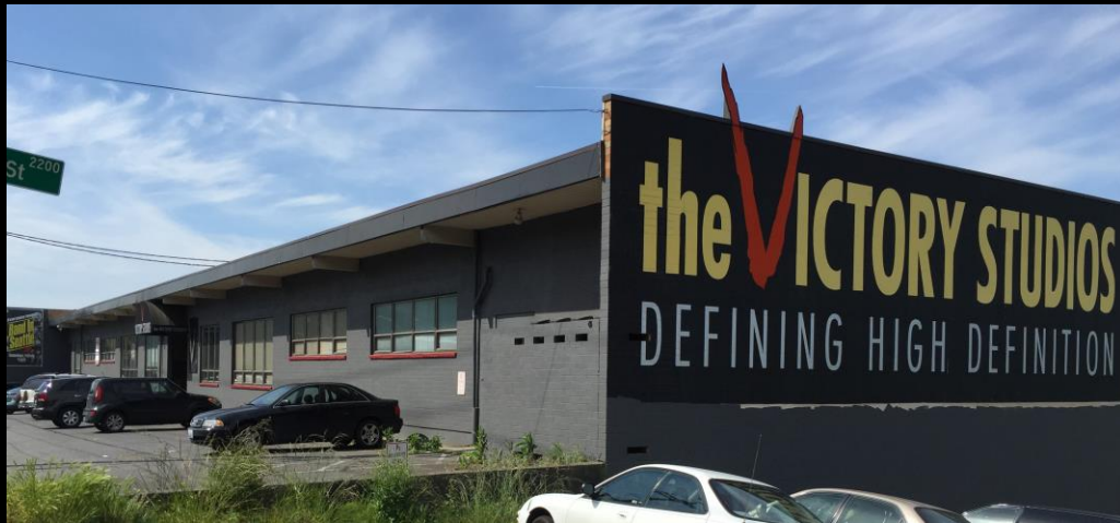
2247 15 th Avenue West, Seattle, WA 98119
